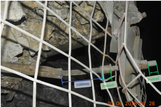
Figure 9: Close-up analysis of one of the Vulcan Bolts that absorbed some of the released energy
