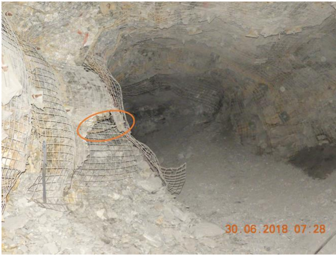
Figure 8: Area subject to seismic event with one of the Vulcan Bolts highlighted.
