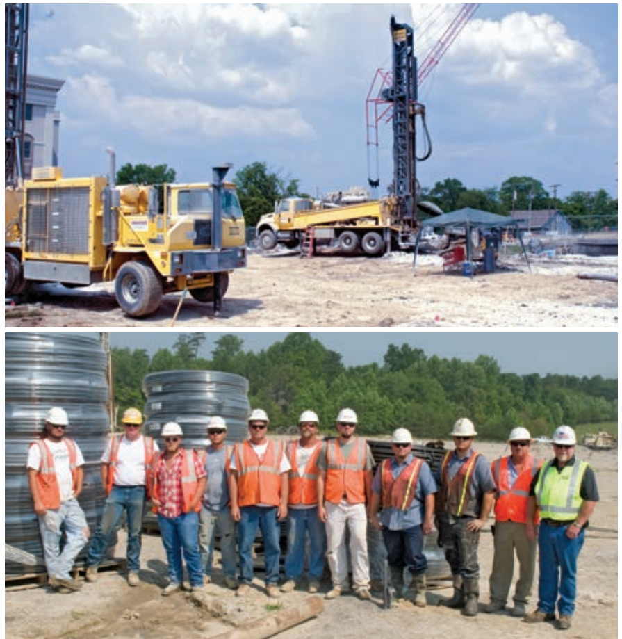
Top: An Atlas Copco T4 and its partnering T3 worked together to drill a hundred 500-foot holes with an Atlas Copco 5 3/4-inch carbide button bit.
