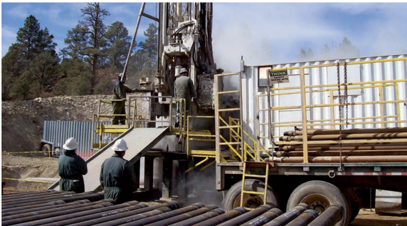
Colorado company uses Atlas Copco's RD20 to efficiently develop unconventional Coal Bed Methane reserves.
