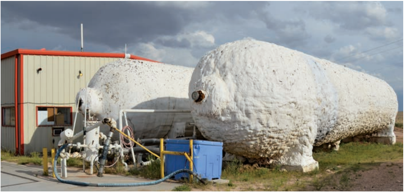
CO 2 is stored in large insulated tanks to keep it in a gaseous form.
