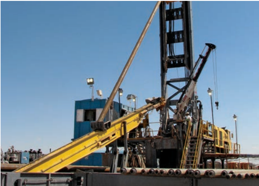
The connection is flawlessly repeated joint after joint as the Predator system's pipe skate lifts pipe to the tilt-out top head of the drilling rig.
