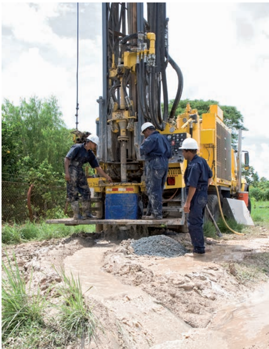
The well pictured above now supports 100 residences with 500 percent growth capacity—just one of the many wells installed with the newly acquired T3W water well rigs to keep up with a surge in the region's market.
