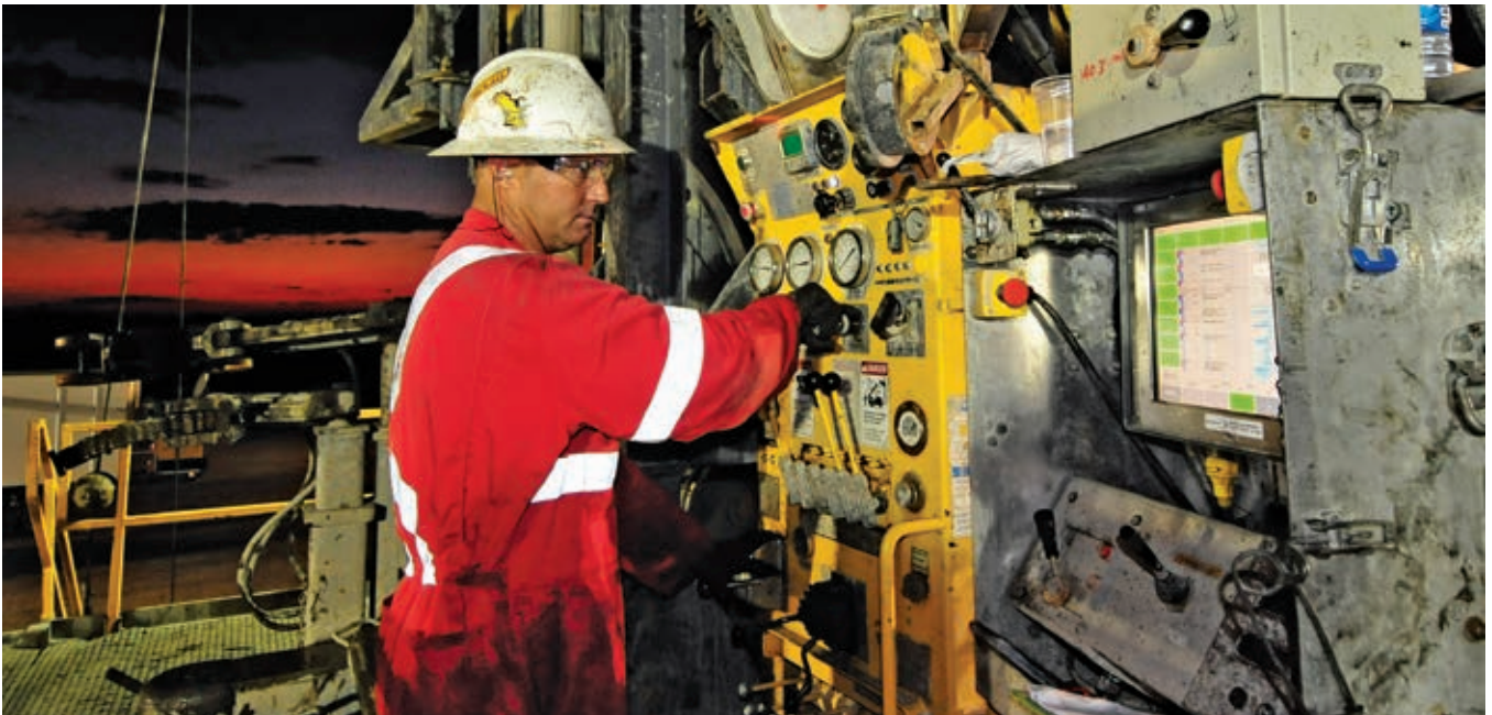
This Atlas Copco file photo shows the ease of pipe handling with the RD20 XC.
