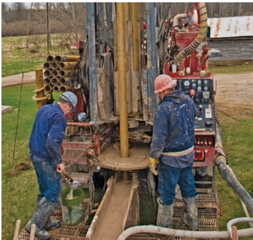
This residential site's existing well tested at 36 parts per billion (0.04 mg/L)—three times the federal limit. However, tests of this replacement well photographed as it was drilled by Leo Van De Yacht's crew resulted in the finding "None Detected."
