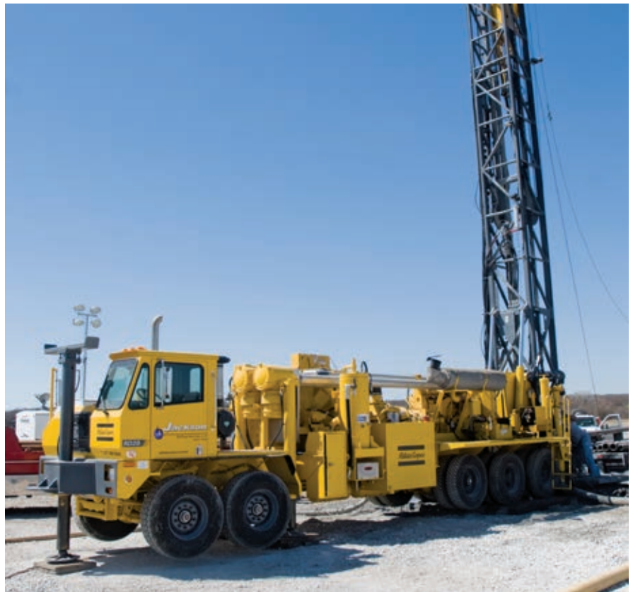
The RD20 XC handles this job's range 3 threaded 9-inch (25 cm) steel casing with ease.
