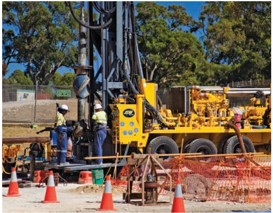
JSW Australia's Atlas Copco RD20 XC is a high-powered compact, hydraulic top-drive rig that sees plenty of work in the geothermal industry.
