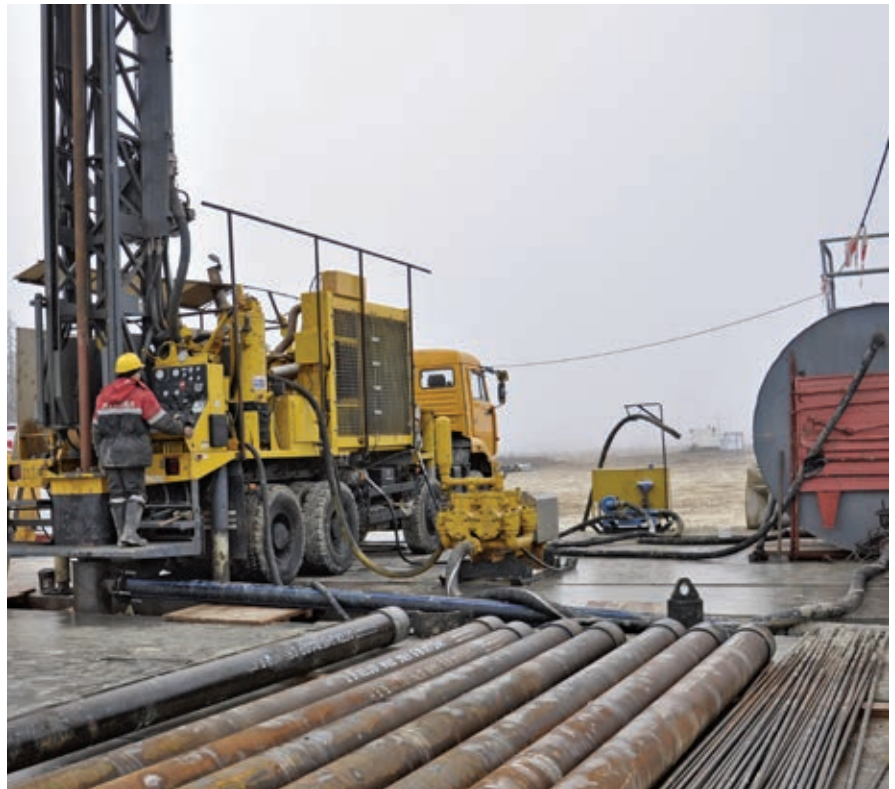
In July 2011, AGR had plans to drill 40 dewatering holes, as well as a few monitoring wells.
