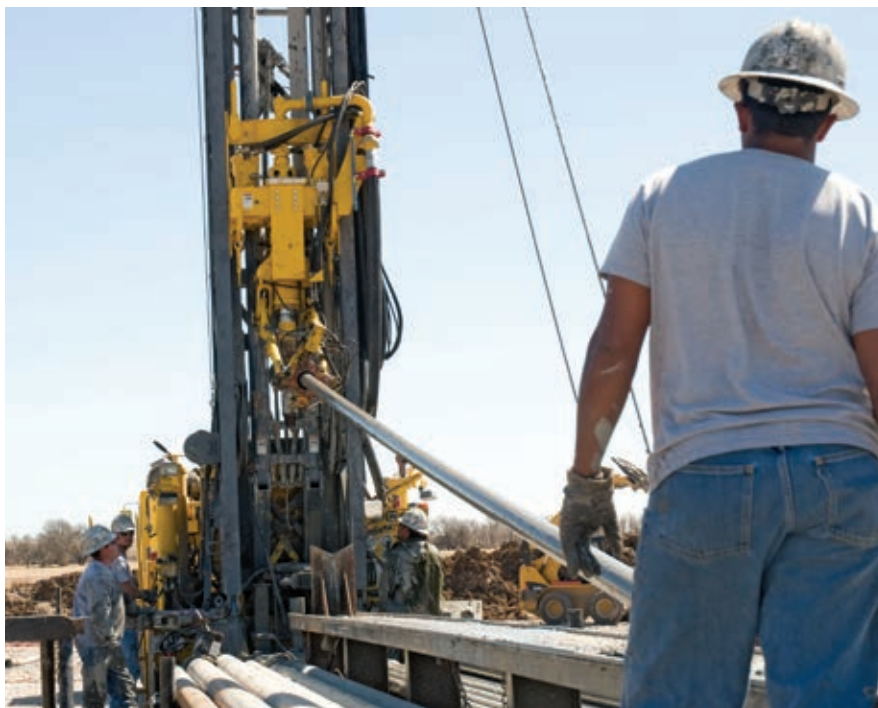
This Atlas Copco file photo shows the ease of pipe handling with the RD20 XC.
