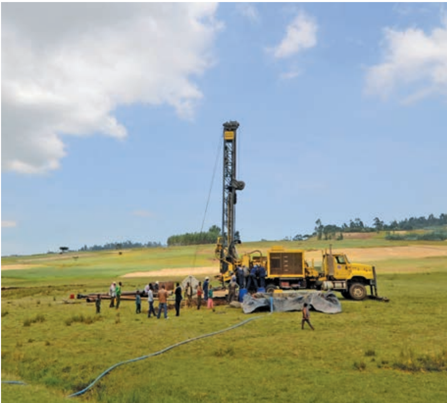
The T3W is shown drilling in the Oromia region.
