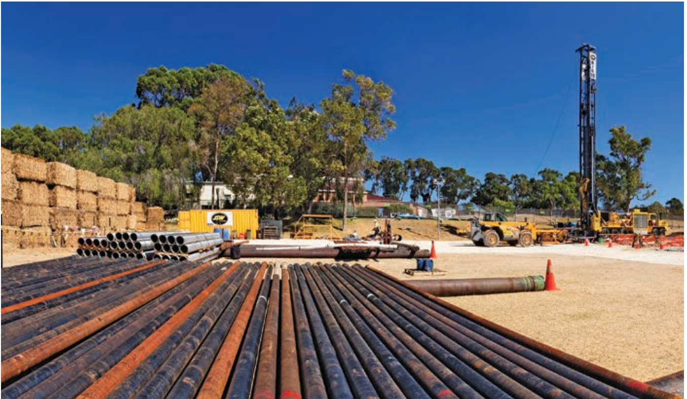
Arguably the world's most successful shallow oil and gas rig in the 120,000-pound class, the RD20 has become a fixture on Queensland's coal basins.
