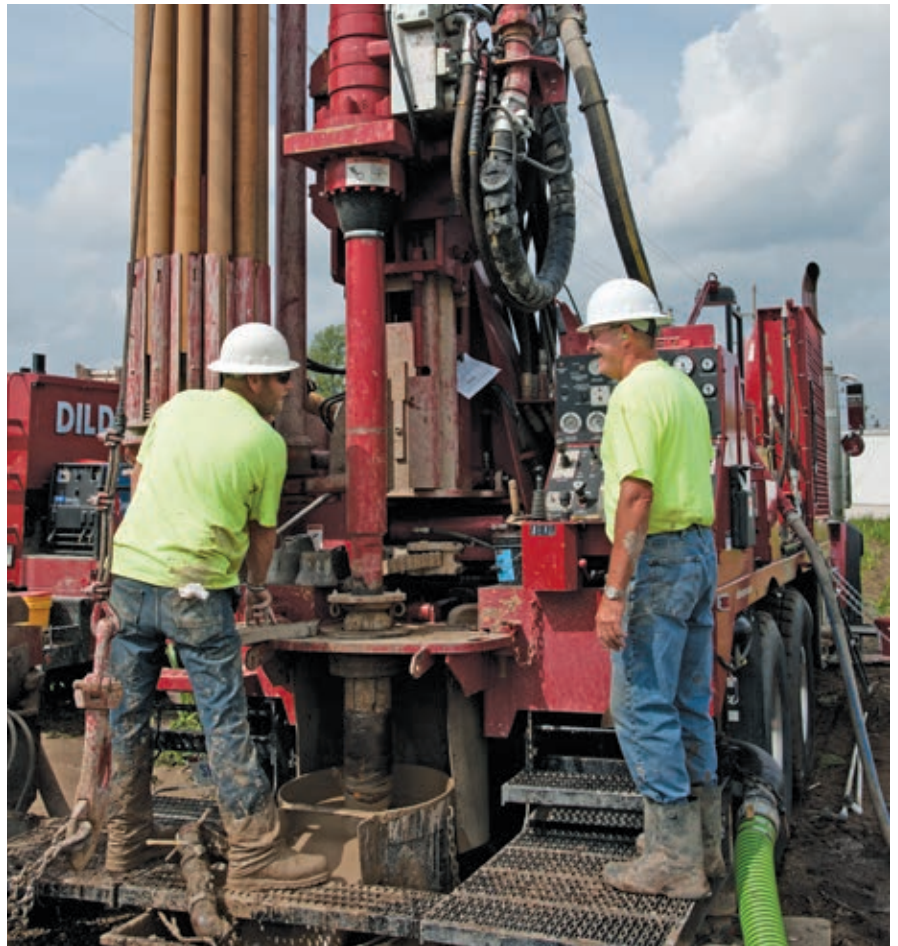
The rig is quiet enough even while drilling, owner-driller Wayne Findlay and helper Mike McCall can easily communicate over the rig's single 500 hp engine.
