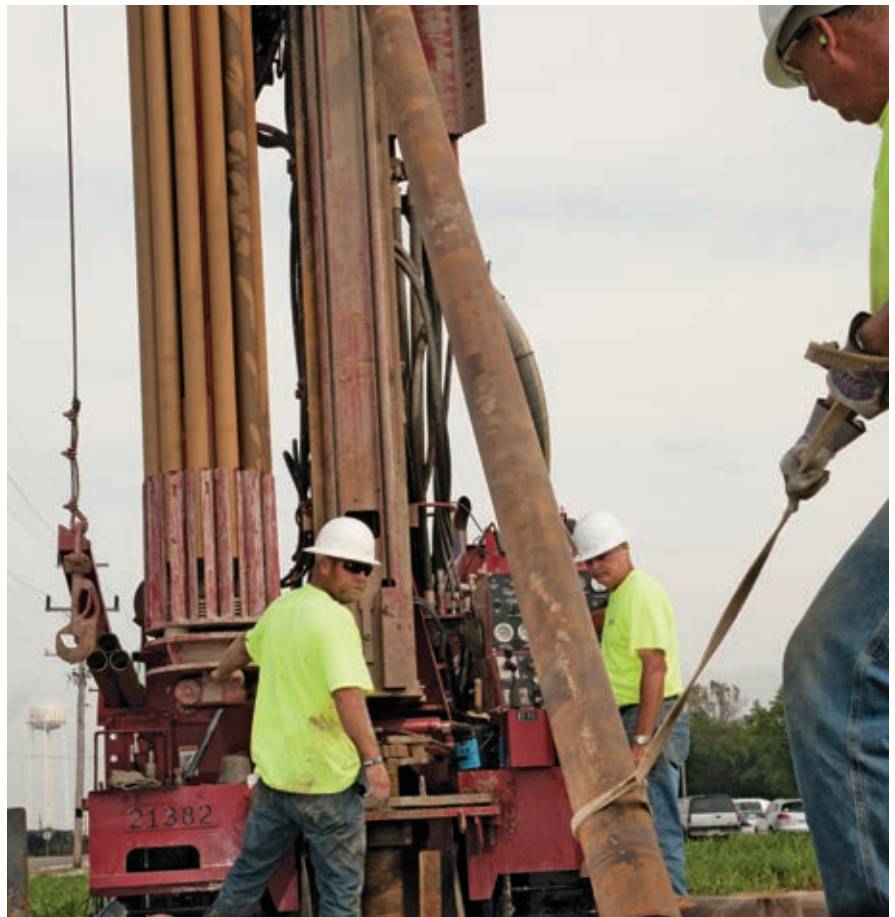
On this irrigation well job Dilden Bros. crews switched deftly from 6 5/8-inch pipe on the trailer to 3 1/2-inch pipe on their 12-rod carousel in moments.
