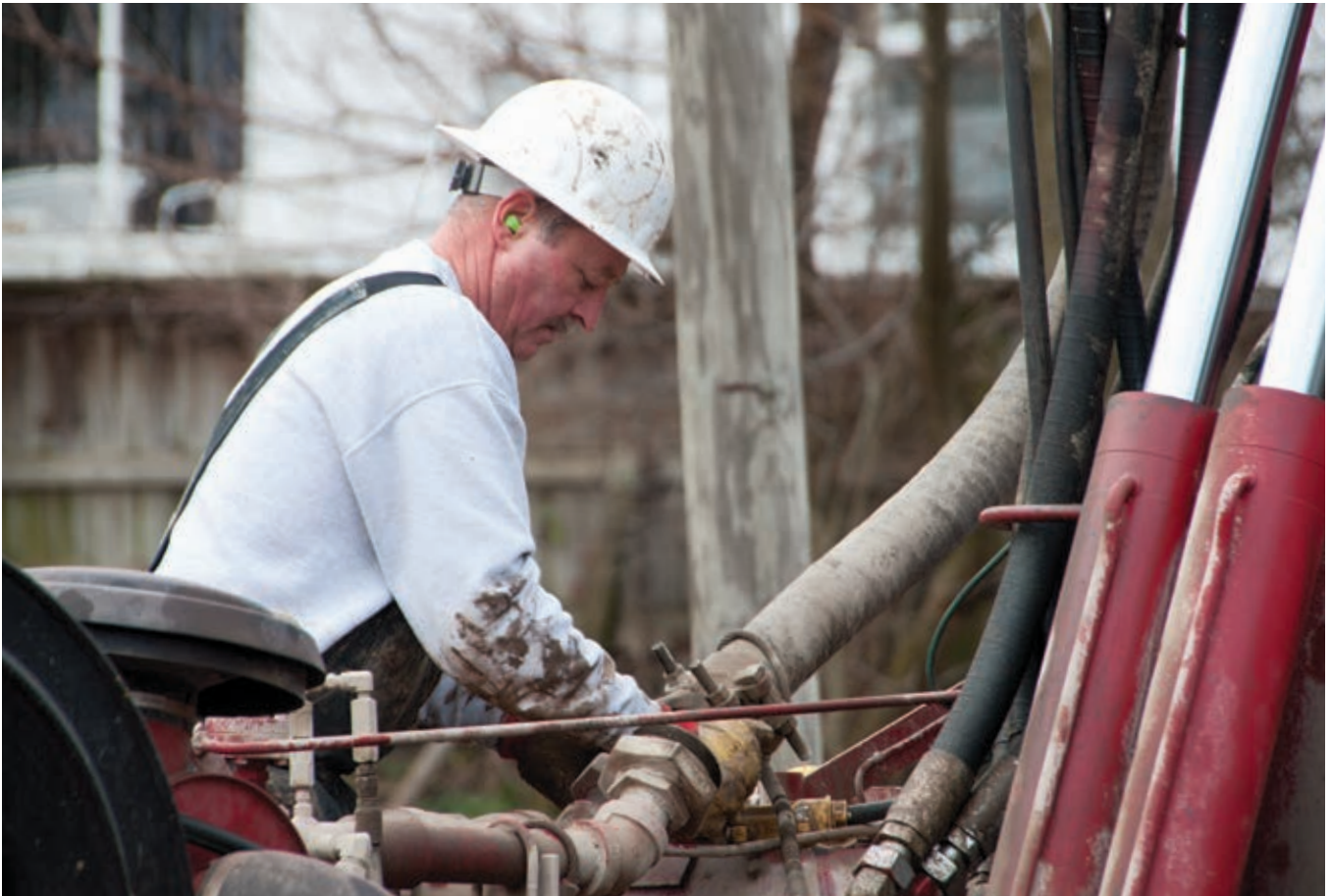
Once a 15-inch socket is created in the limestone, Wayne Findlay switches from mud to air to put the QL 120 to work on the Muncie municipal well. With a 15-inch concave bit, rate of penetration was anywhere from 10 to 15 inches per minute in fractured limestone.
