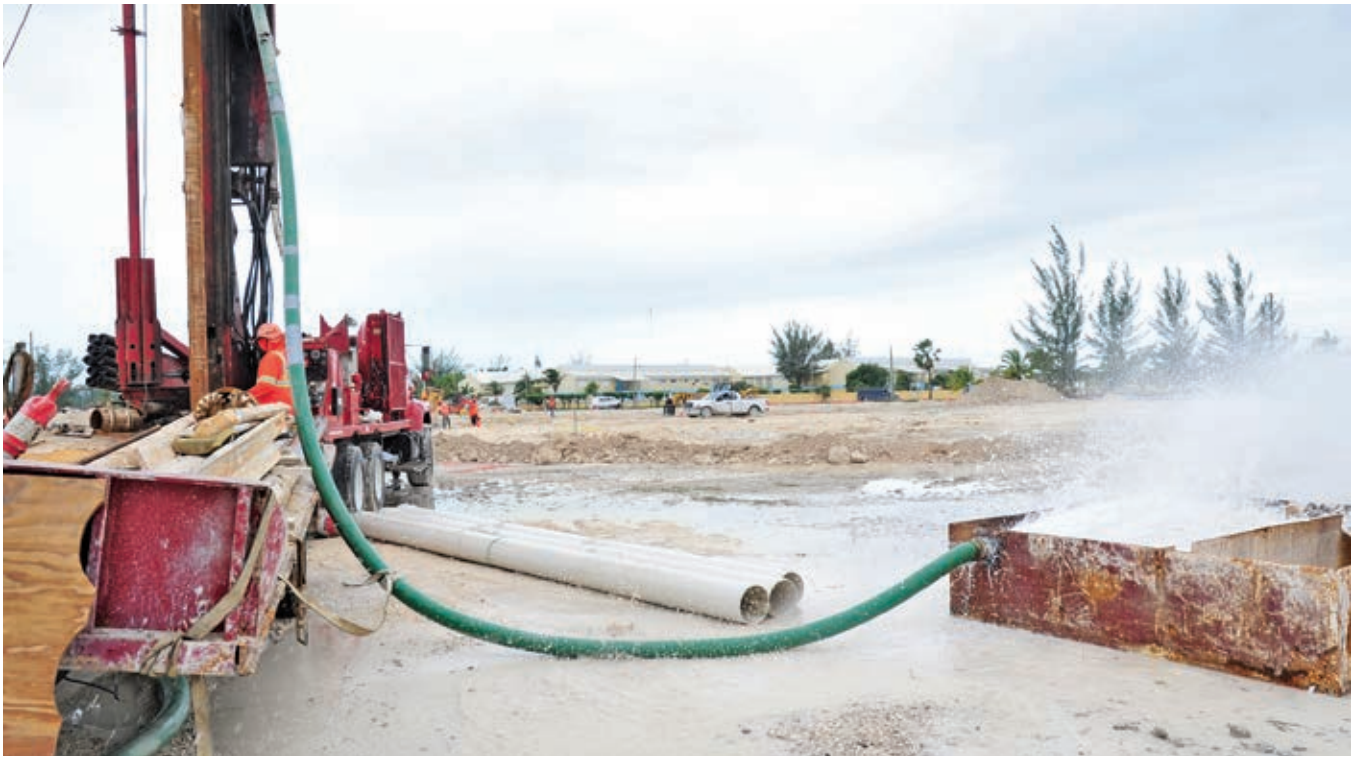
Cuttings from the discharge line are captured in a steel box so they can be hauled away or disposed of easily. Attaching the discharge line to the box anchors the line and diverts water away from the work area.
