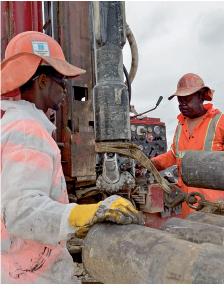
Joseph "Spike" Mather just finishes hooking the wench line for Driller Vernon "The Bear" Moss to pull back to the pipe trailer.
