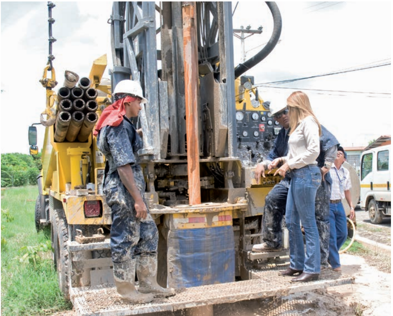
Workers near completion of the numerous wells of an IDAAN initiative talk with Nancy Gaitan, IDAAN Maintenance Manager on site. Geology throughout the area required both mud and air drilling methods to penetrate the various layers of heavy loam and clay, consolidated sandstone and igneous rock.
