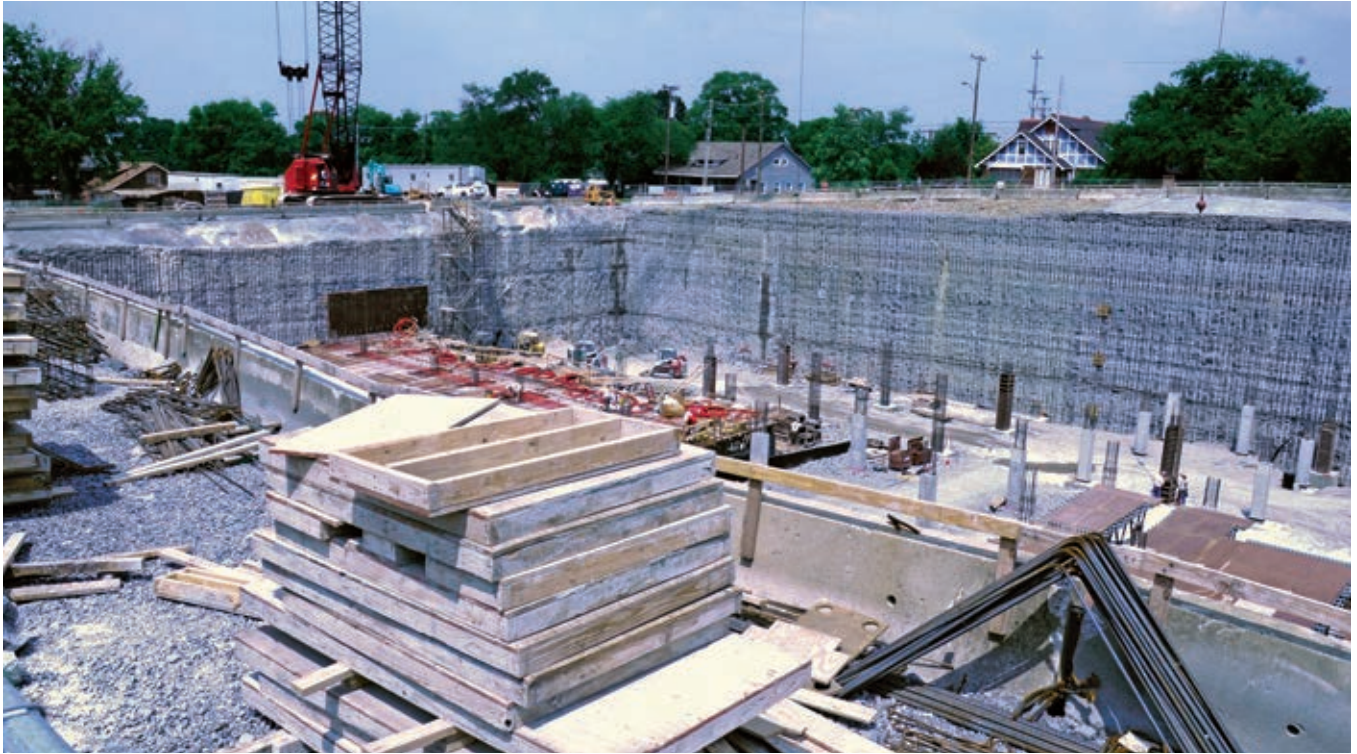
The geothermal loop field was installed alongside the 60-foot (18 m) excavation for the College of Law's new facility. Incidentally, the perfectly parallel bores on the excavation's walls represent the signature line drilling also done by Mid-State with an Atlas Copco T4W but with a 6 1/2-inch bit.
