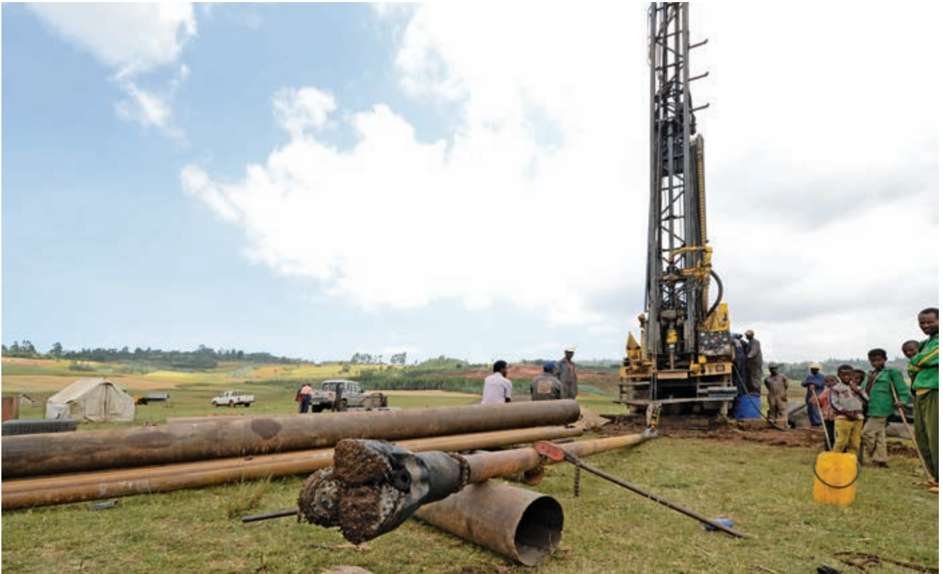
Along with the Atlas Copco T3W, crews use Atlas Copco down-the-hole hammers and a tricone bit when necessary.
